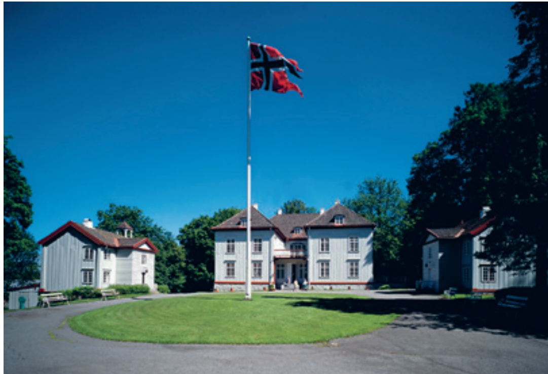
[3.6] The Eidsvoll building of 1770, Eidsvoll.
