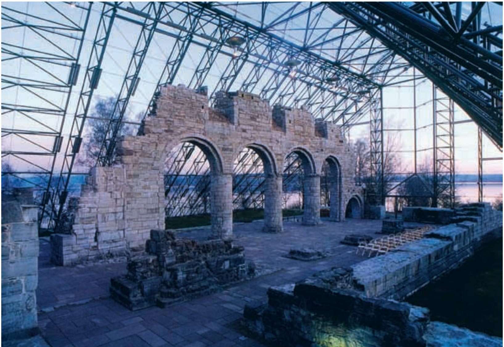
[3.4] Cathedral Headland. Hamar (Lund + Slaatto Architects AS)
